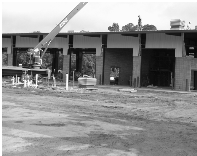
New Fleet Management Facility under construction.
