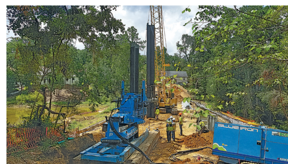
Centerville Trace Stormwater Improvements
