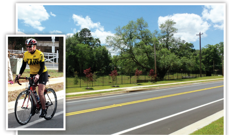
Buck Lake Road Reconstruction Project
