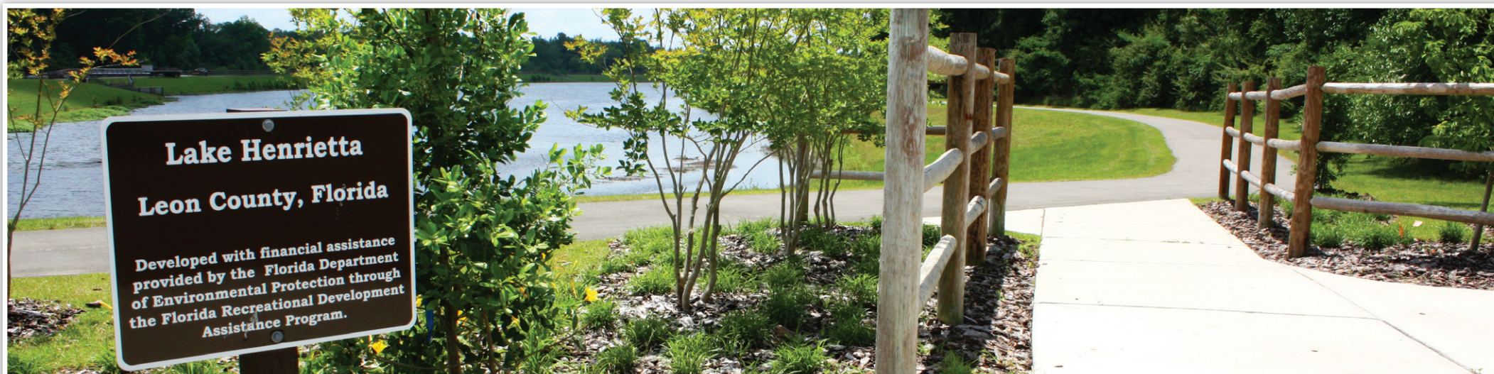
Lake Henrietta Park – Stormwater Pond
