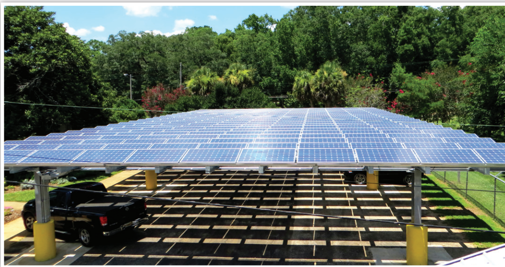
Leon County Cooperative Extension Net-Zero Facility
