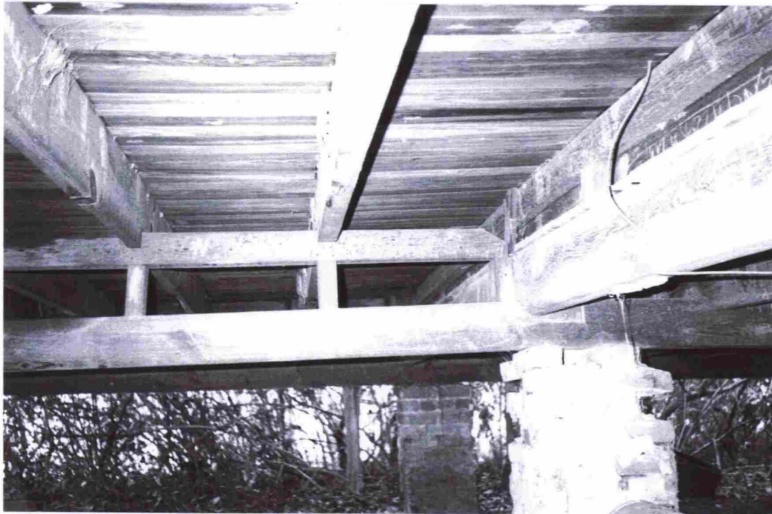
Floor framing under addition on west end of school..
