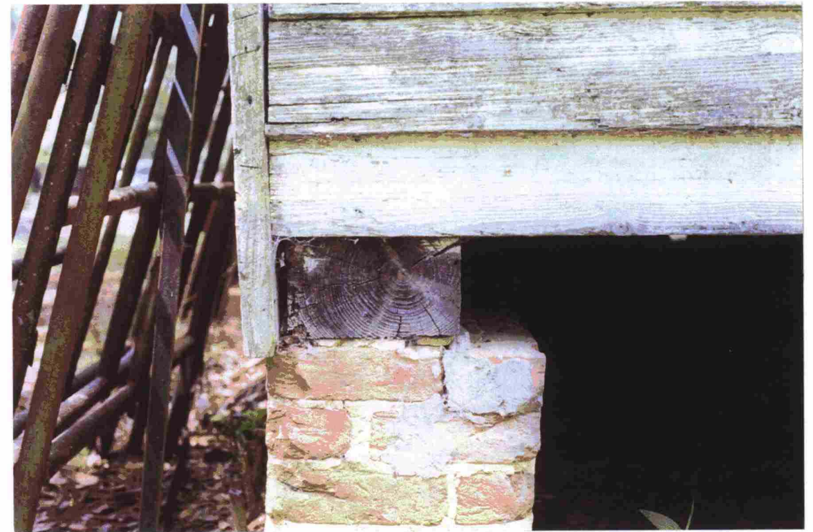
Southeast corner of original structure. Note 6"x 8" perimeter beam set with the 8" dimension bearing. Perimeter beams are typically set with the short dimension down. Notched joists run perpendicular.
