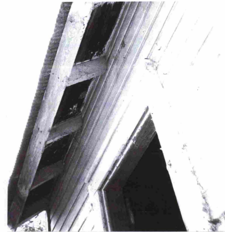
The roof rafter end detail at the addition on west end of schoolhouse.
