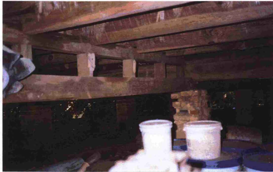
The extended center beam under the west end addition to the Lake Hall School..
