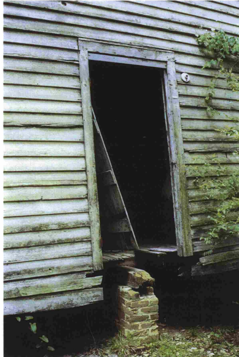
The Lake Hall School. Primary entry door. Note door in opening, no longer attached to frame. Severe deterioration present at perimeter frame in north-south direction. Stairs once located here Have been removed.
