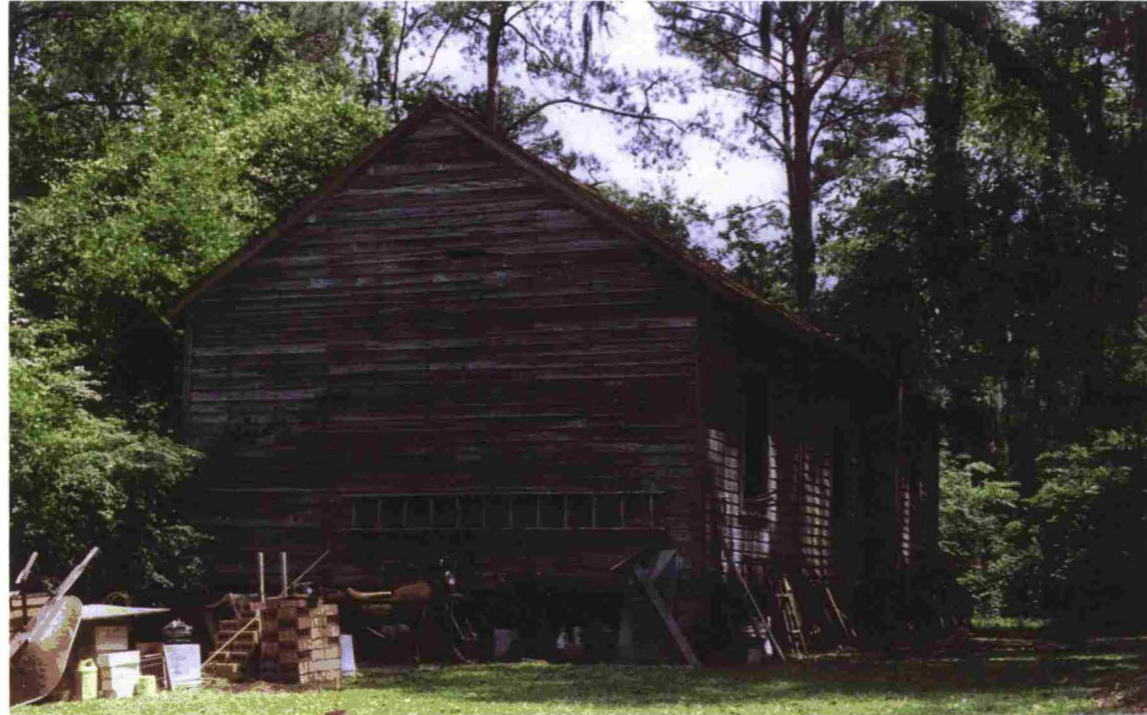
The Lake Hall School. Currently used as a Storage Building
