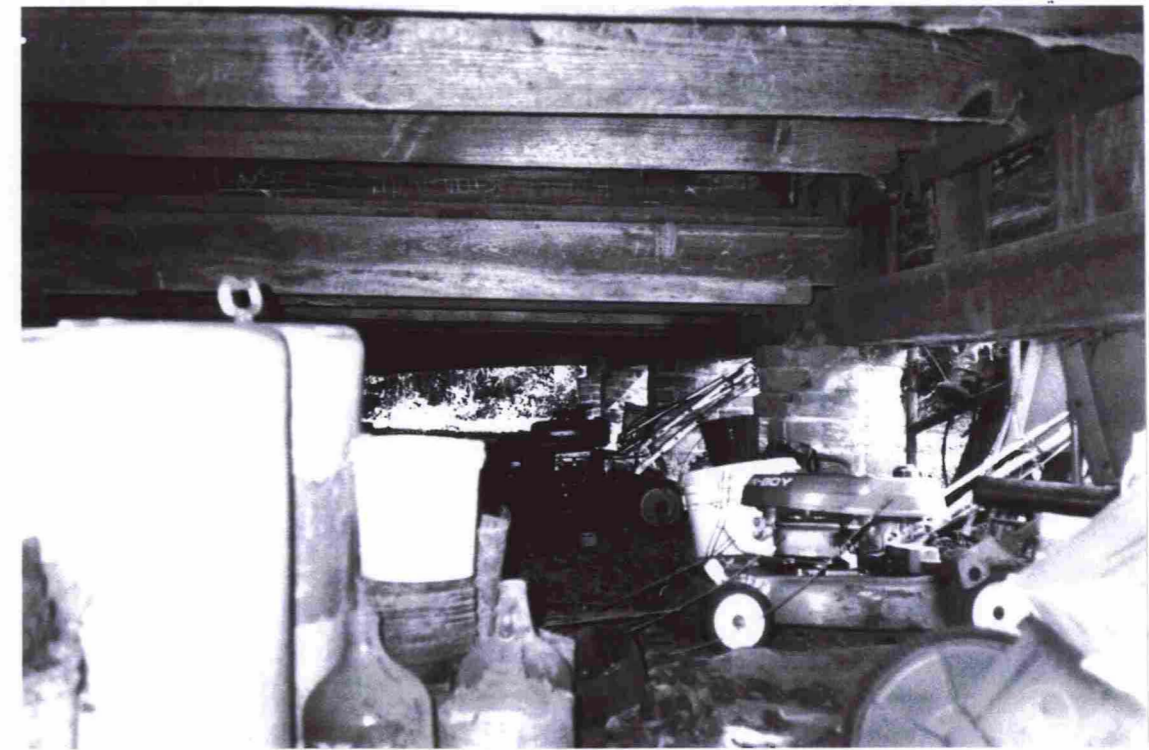
Perimeter of structure on south side at intersection of original structure and addition
