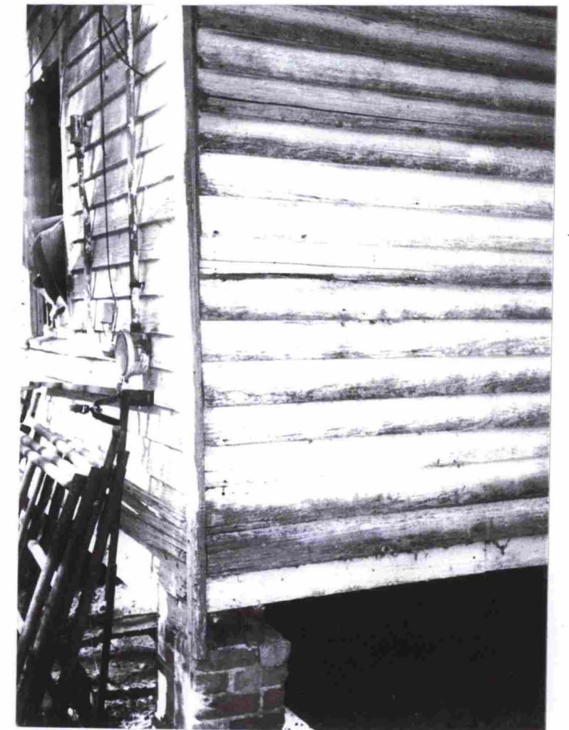
Electrical meter suggests the building had electric lighting.
