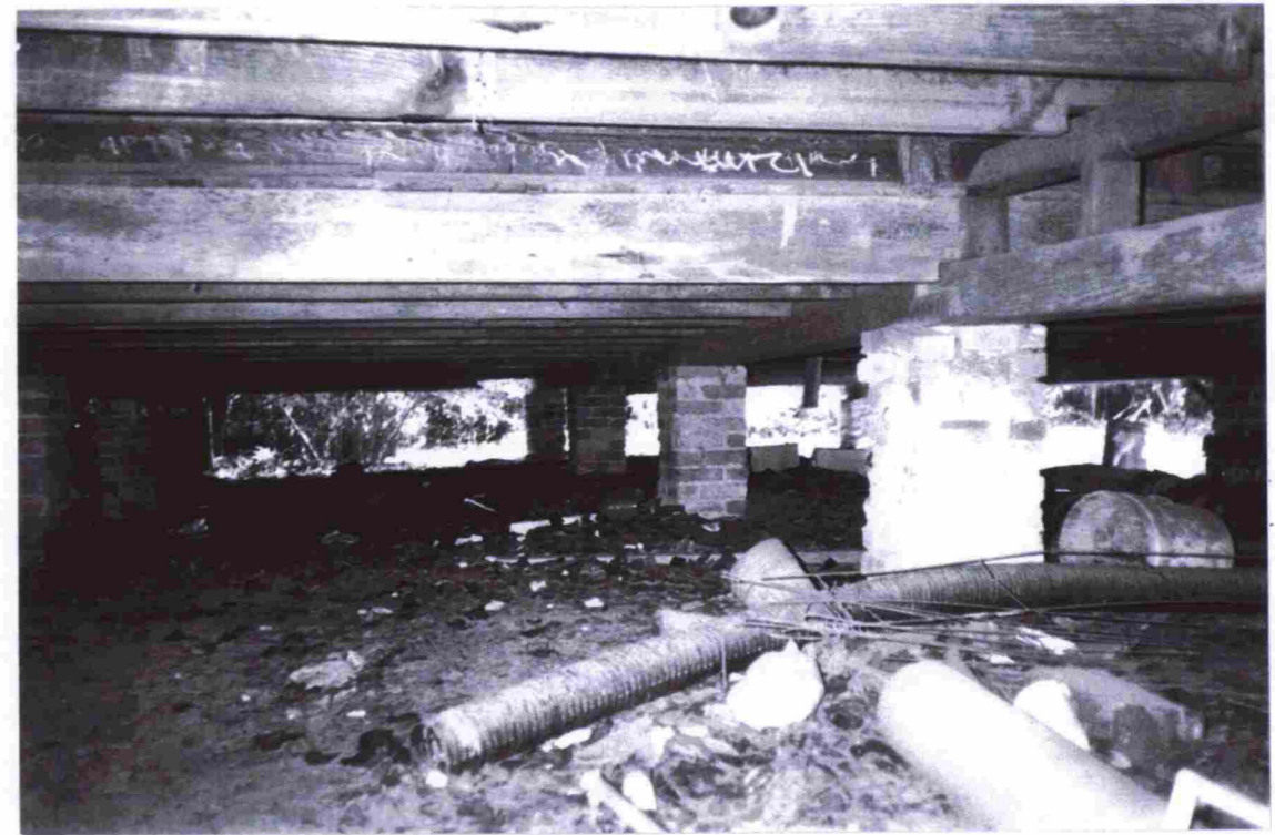
Floor framing at the center pier at intersection of original structure and addition.
