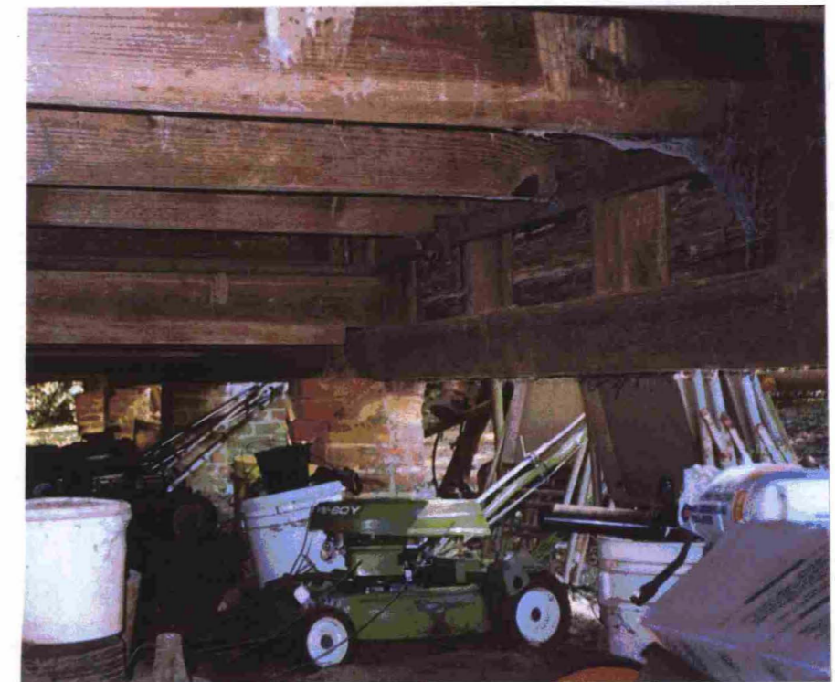
Photo of perimeter at addition on west end. Lower beam is the extension of original school. This provides platform raised above former level of school.
