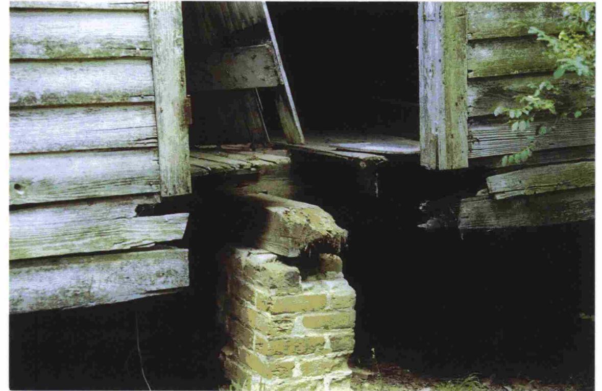
Close up view of former school entrance and deteriorated perimeter beam. Note original pier form and construction. Door and window frame details and construction clearly discernable.
