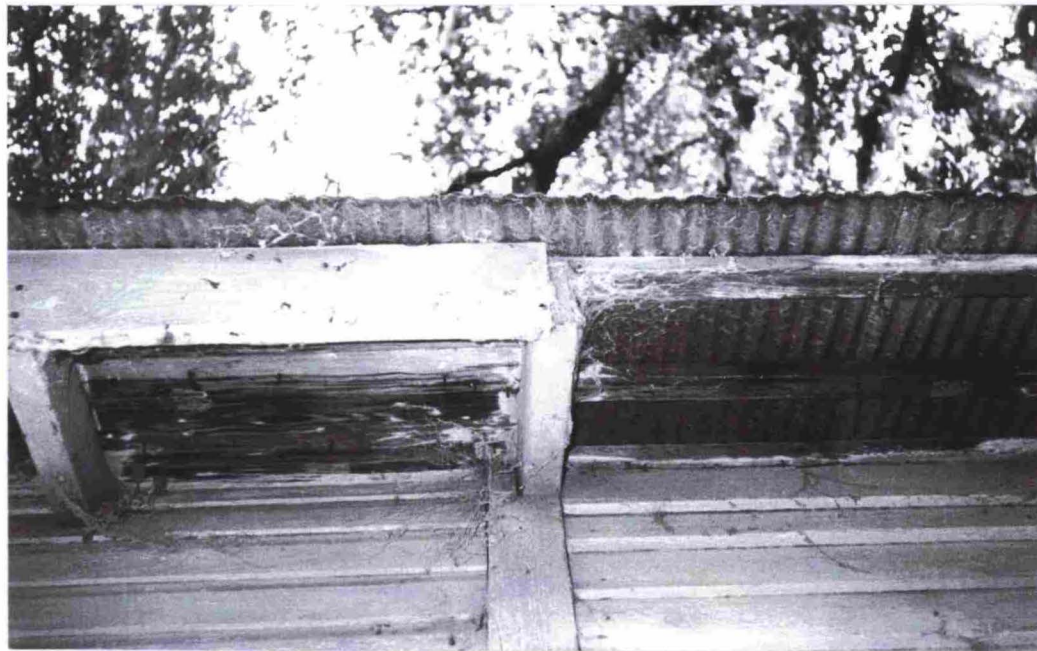
The change in roof sheathing and framing between original and addition. Note the roof is sheathed at the addition and uses purlins at the original. This suggests a different roof material was also used on the original.
