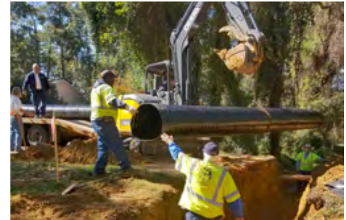
Crews place drainage pipe in Killearn Lakes
