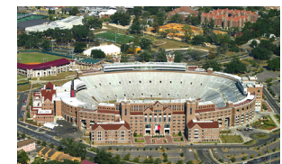
Florida State University Academic Center Multi-Purpose Education Facility 9 stories/600,000 GSF $110,000,000.00 Tallahassee, Florida
