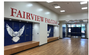
Fairview Middle School Renovation & Addition 106,000 GSF $20,000,000.00 Tallahassee, Florida
