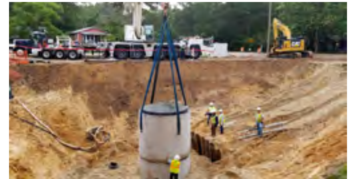
Woodside Heights Septic to Sewer project
