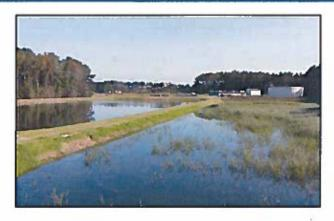
advanced treatment through the constructed wetland. In the design of this system, several P-k-C\* and TIS computer models were created to determine the percolation rates, treatment efficiency, and size of the additional pond(s) required to meet a future flow rate of 0.5 MGD. System monitoring has found a nearly 85% reduction in nitrogen and phosphorus.
