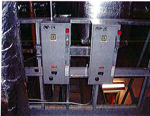
Constant speed pump controllers to be replaced with variable speed units.
