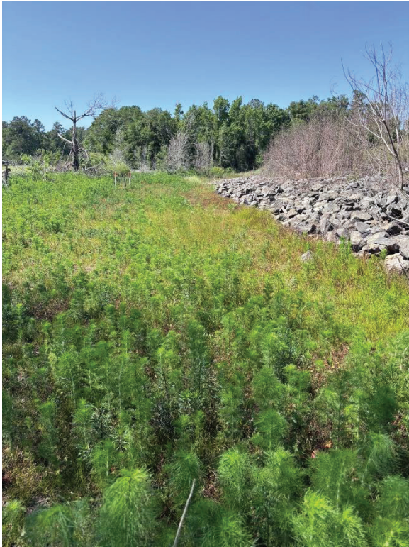
View along Downstream Toe Southwest of Outfall
