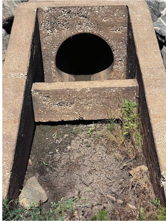
View of 24-Inch Outfall Looking Upstream
