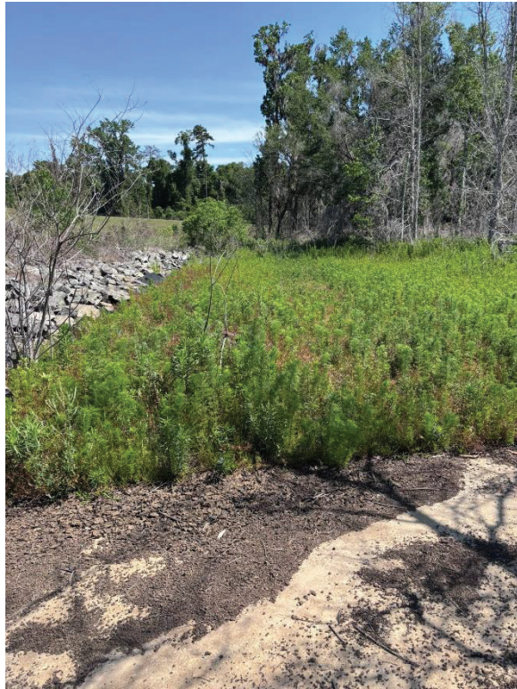
View along Downstream Toe Northeast of Outfall
