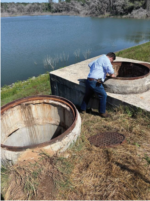
View of Vaults from Dam Crest
