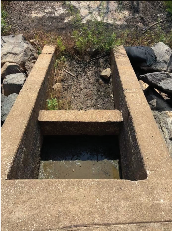
View of 24-Inch Outfall Looking Downstream
