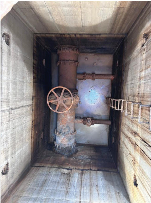
View of Vault for 24-inch Pipe Valve
