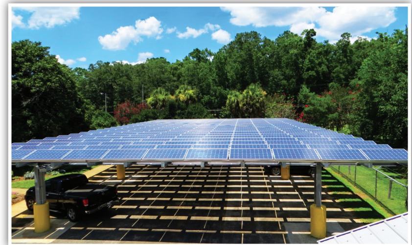
Cooperative Extension Net-Zero Facility
