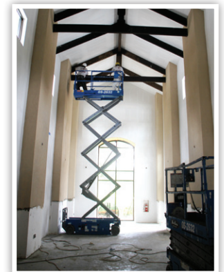
Eastside Branch Library
