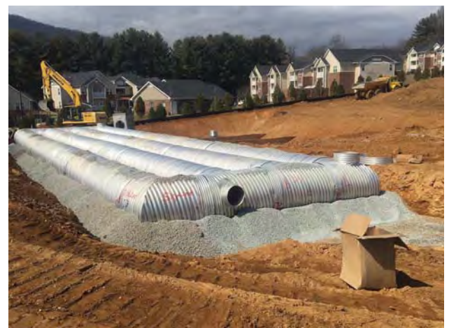
BENEATH PARKING AREAS - PIPING
