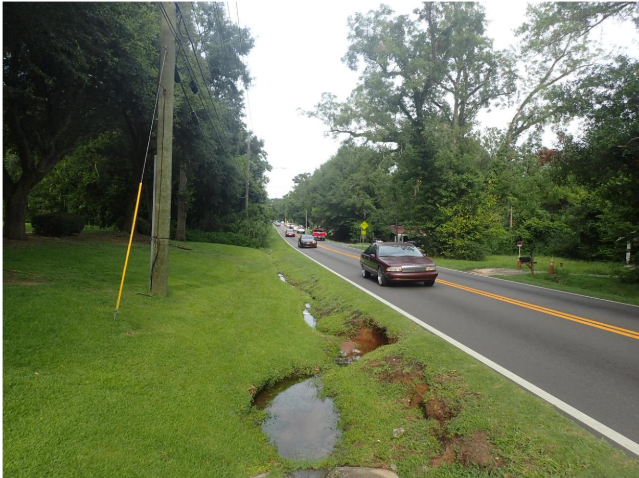
Figure 8. Slope Erosion Caused By Stormwater Runoff along Tharpe Street
