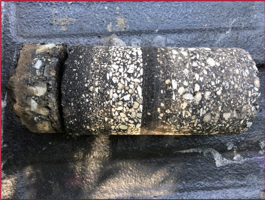
FIGURE 5A: PHOTOGRAPH OF PAVEMENT CORE AT P-1
