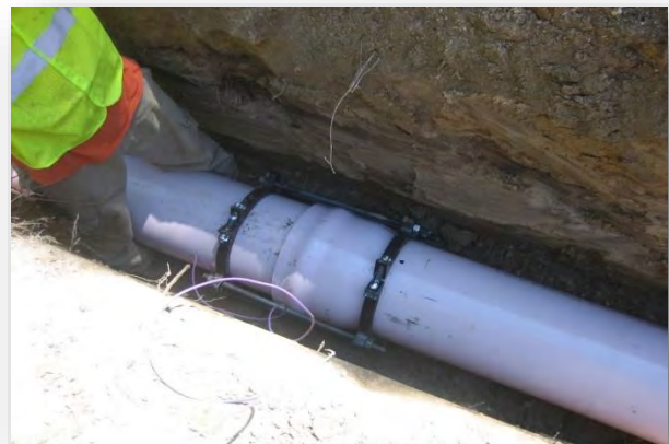
Reuse Forcemain Construction
