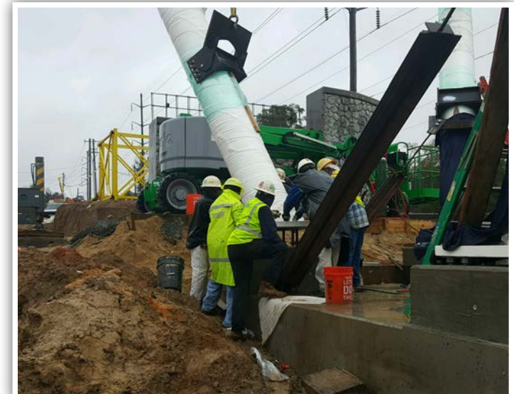
Bridge pier installation at Capital Cascades Crossing
