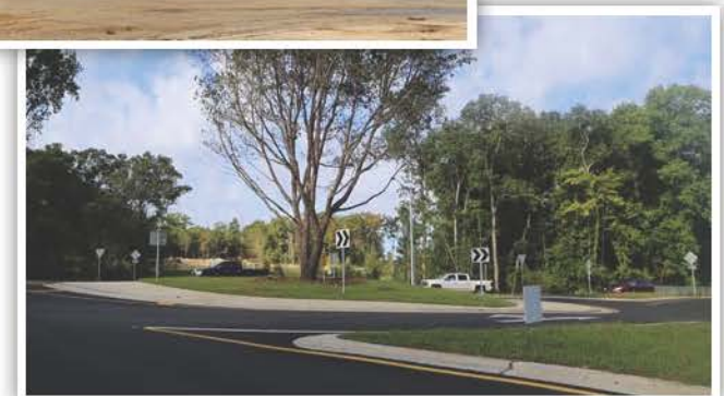
Kinhega Roundabout Improvements
