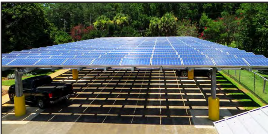
Leon County Net-Zero Facility
