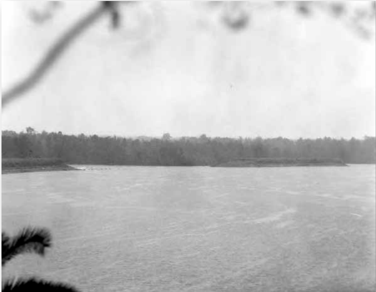
Figure 34: 1957 Break in Jackson Bluff Dam. 103
