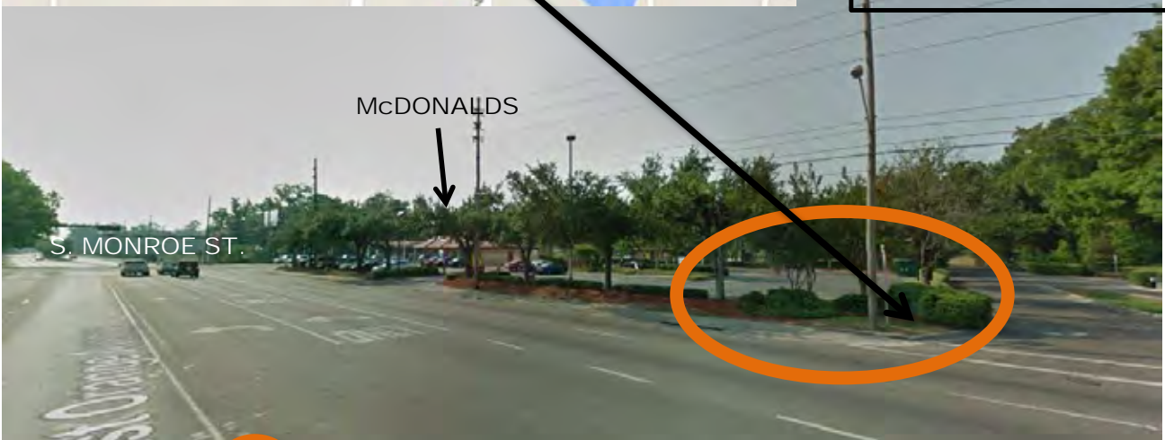
SS VH 3 Vehicular directional, Orange Ave. EB at S. Monroe St. southwest side
