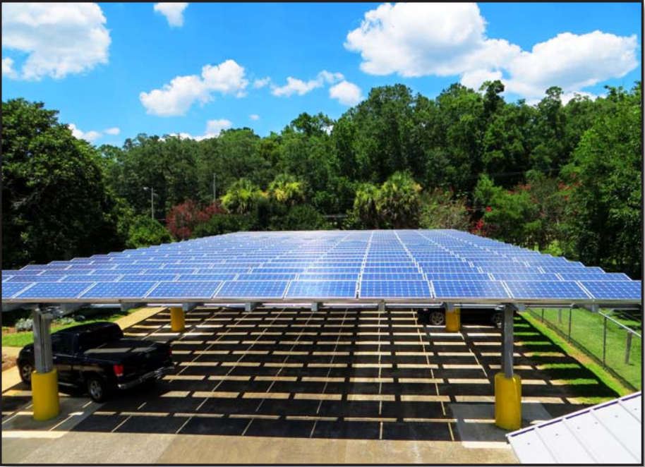
Leon County Net-Zero Facility
