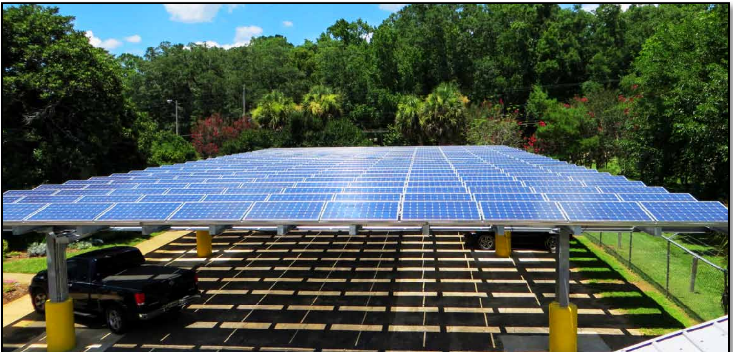
Leon County Cooperative Extension Net-Zero Facility
