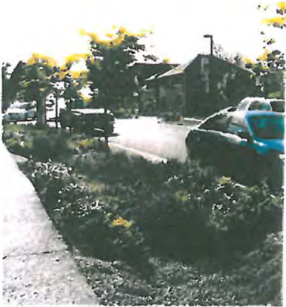
In Seattle's High Point neighborhood, roadside bioswales collect and filter stormwater, create a park-like feel and improve pedestrian safety.
