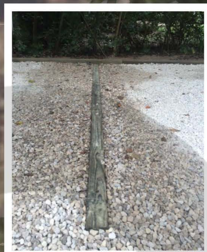
PARKING SPACES DELINEATED WITH WOOD BUMPERS (4x4x20 TIMBERS)
