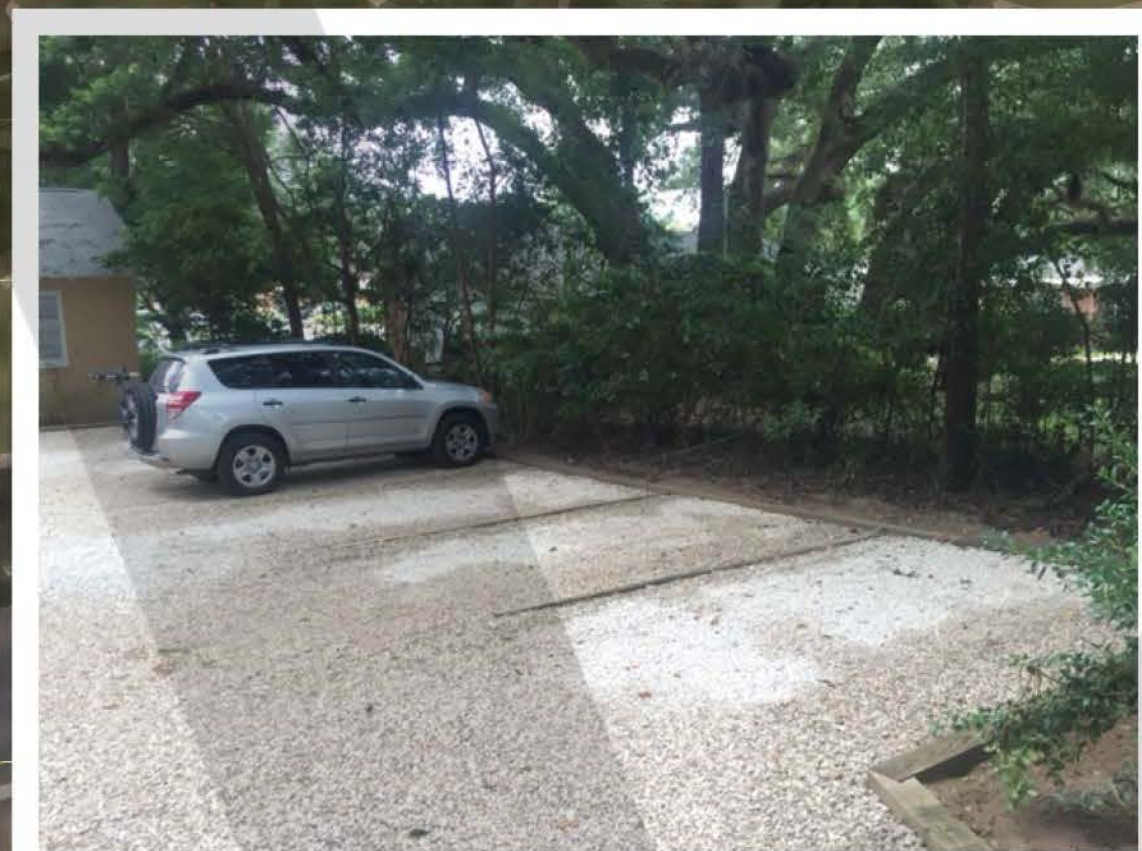
PARKING AREA WITH SUB-BASE SURFACE COMPACTED
